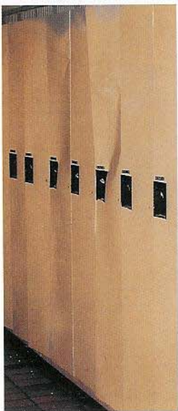
Original condition of the school's lockers.
